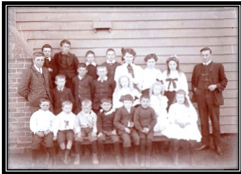
The First School. Fred Stokes pictured leaning against the brick chimney
